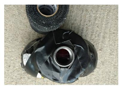
Next wrap the whole thing with Duct or Gorilla tape in all different directions. Do NOT tape over the opening on the bottom of the flange.
